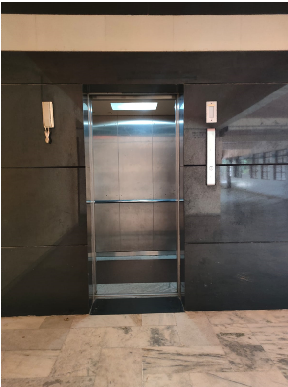
BOYS HOSTEL ELEVATOR
