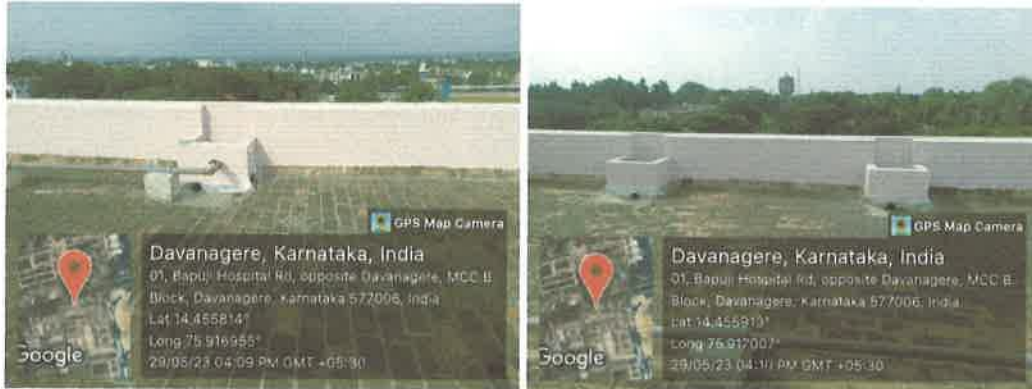
Photos 2 showing Roof top rainwater collection
