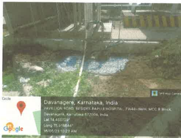
Photo 4 shows bore well recharge
